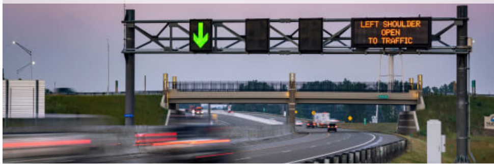
Hard Shoulder Running
