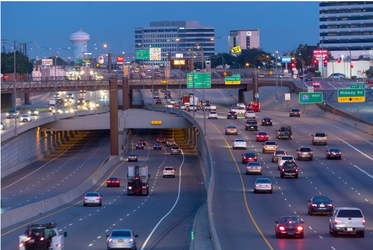
Figure 14: Example of Managed Lanes – I-635 in Dallas, TX
