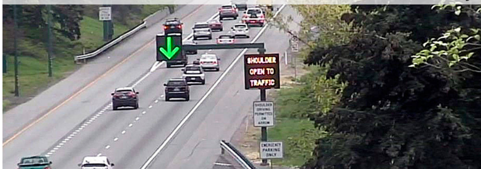
Hard Shoulder Running
